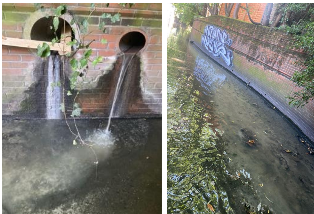
Figure 3. Outfall scoring 20 identified on the lower Brent during ZSL Outfall Safari (Credit: ZSL).
