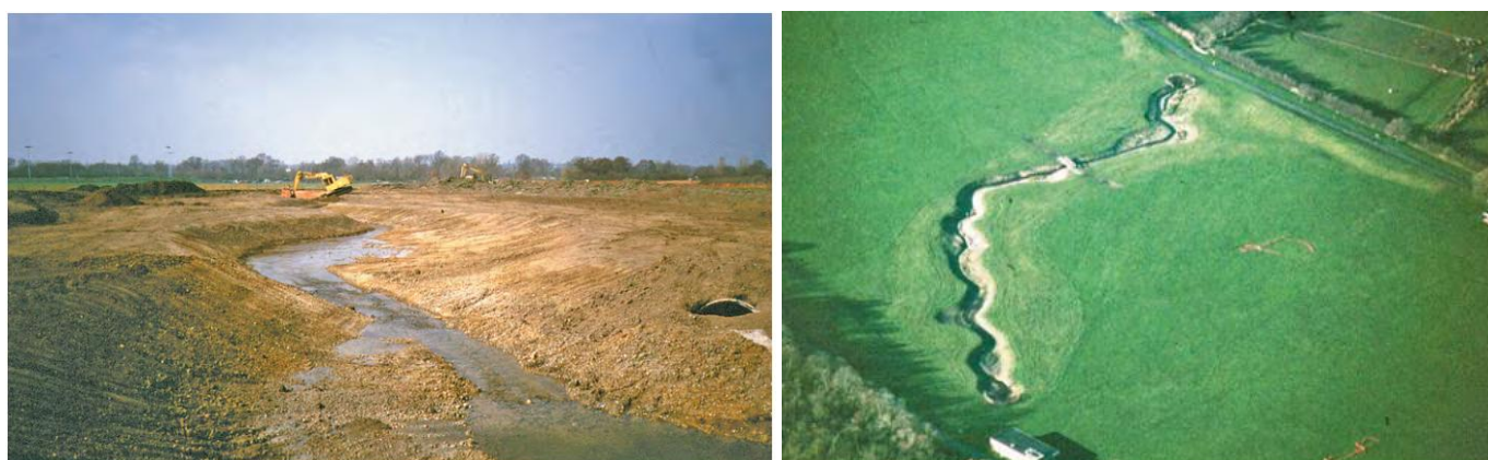
Figure 11. Daylighting the river Ravensbourne through Norman Park. Left photo shows the severed culvert still visible. Right photo shows an aerial view of the re-meandered course (Photos taken from The River Restoration Centre 2013).
